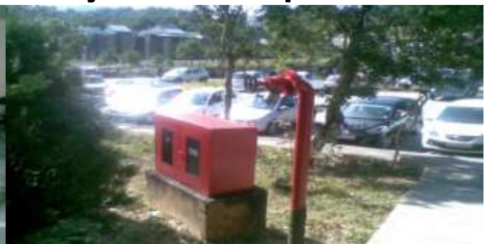
Fire Extinguisher and Hydrant Installed In the Hospital area
