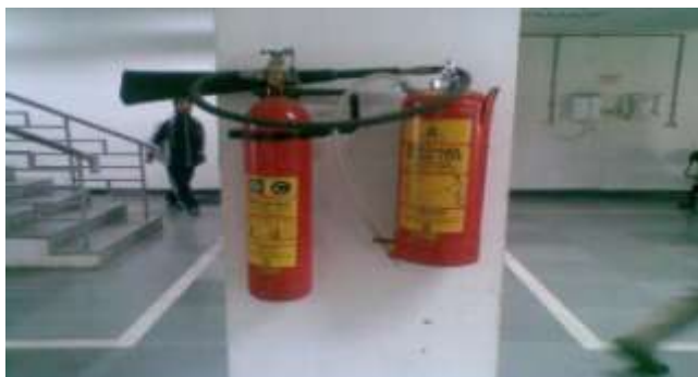
Fire Extinguisher and Hydrant Installed In the Hospital area
